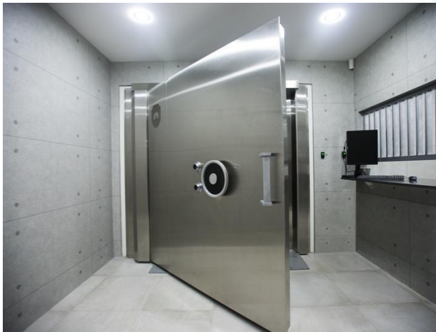
2.5 ton Class I vault door leading into the silver vault at The Safe House, Silver Bullion's subsidiary
